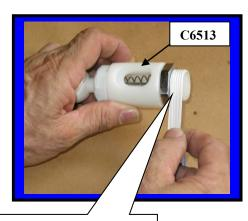
Applying Teflon Tape to **Faucet Body** before installation
