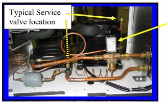
Valves automatically open on pressure increase, close on pressure decrease. <u>Adjustment:</u> To raise valve opening point, turn adjusting screw, on top of valve, counterclockwise. To lower operating point, turn clockwise. Opening point of valve should be raised just enough to cause valve to close when compressor is off.
