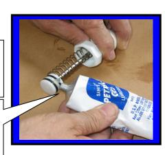
Installing Plunger assembly C6513P into faucet body
